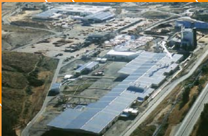
Aerial view of our new state-of-the-art Nueva Aldea plywood plant, north of Concepcion, Chile
