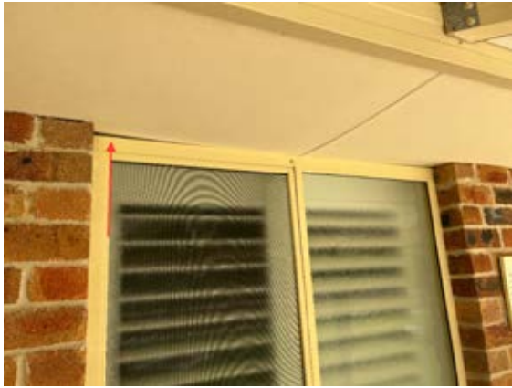
Settlement has created a gap between eave and window.
