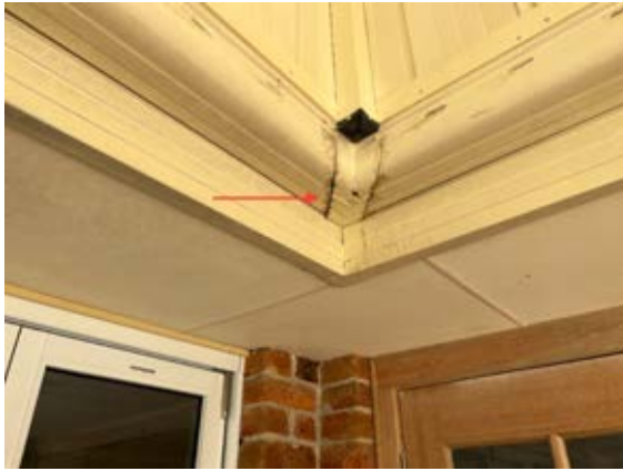
Area where susceptible of leaking.
