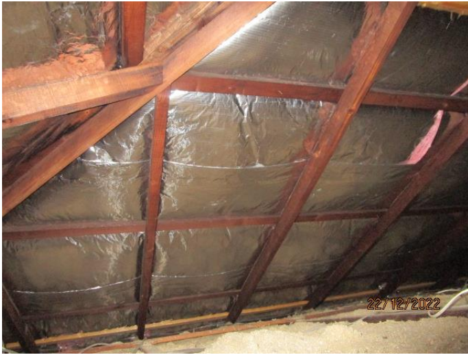
64. The roof structure is in very good condition.
