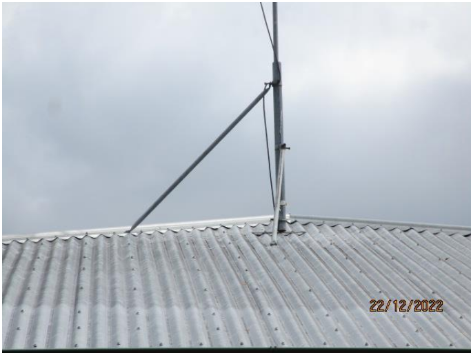
18. The roof is in very good condition.
