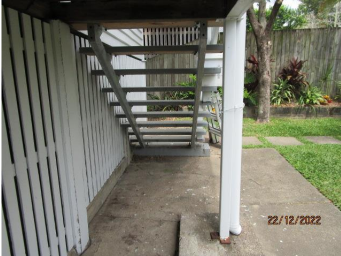
25. The base of the front column has rust and requires treating against rust. The stairs are in very good condition.
