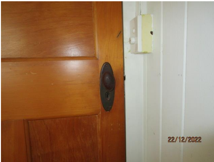
38. The entry doors function.
