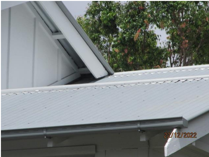
66. The roof is in very good condition.
