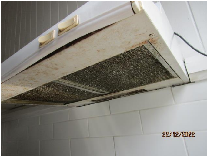
The range hood light requires replacement. The grease catcher requires repairs or replacement. The front panel does have a buckle.
