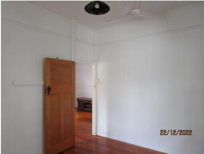
37. The entry doors to the bedrooms function. The bedrooms require interconnected smoke alarms.
