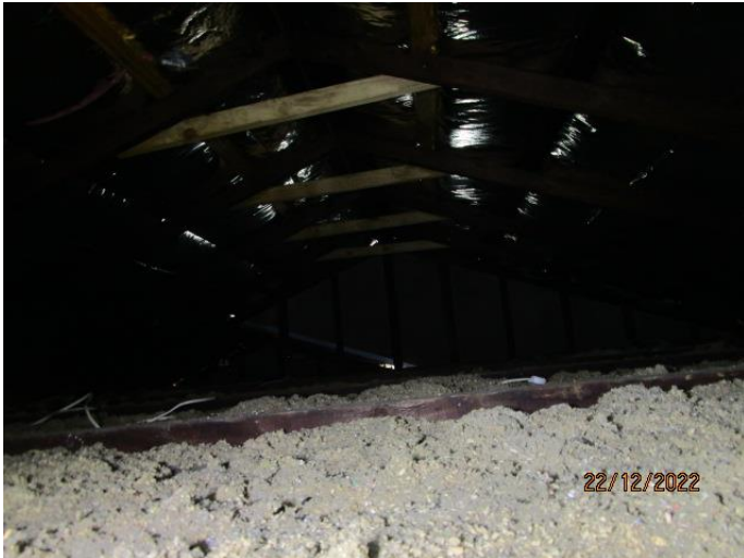
63. The ceiling is also insulated.
