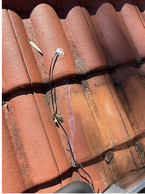
Photo Ref #29: There is one cracked tile repaired with silicon. This should be monitored as silicon will deteriorate
