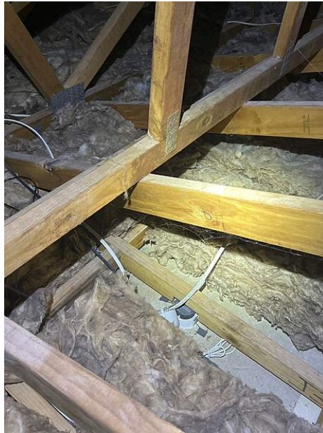
Photo Ref #19: There has been improper modifications to the bottom cords for light fittings in areas. Additional strengthening should be installed to prevent structural integrity to the roof framing.
