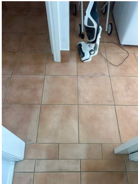
Photo Ref #14: There are areas of drummy tiles to the laundry floor. These may come loose and/or crack over time.
