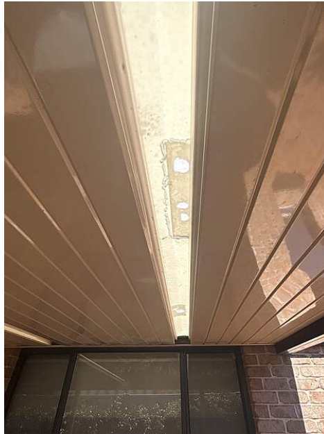
Photo Ref #25: There is evidence of patching to the roofing sheets
