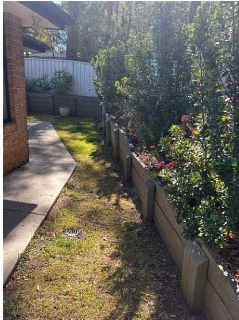
Photo Ref #26: The timber retaining wall is out of vertical alignment in areas. This should be monitored for further deterioration and repaired/ renewed as necessary.
