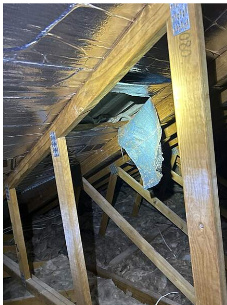
Photo Ref #21: The sarking is torn in several areas. The affected areas
