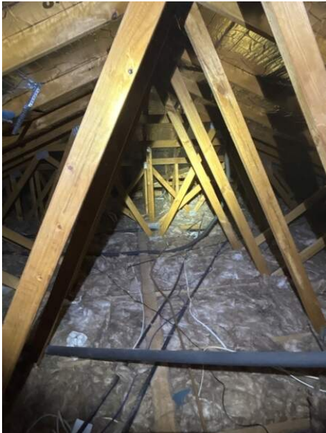
Photo Ref #18: The roof is trussed construction with sarking beneath the tiles and insulation to the ceiling sheeting.
