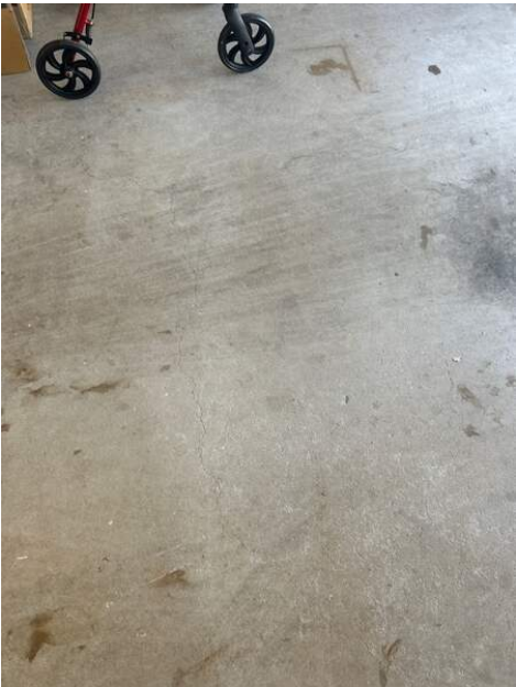
Photo Ref #23: There is minor to moderate cracking to the garage concrete floor. This should be monitored for further cracking.
